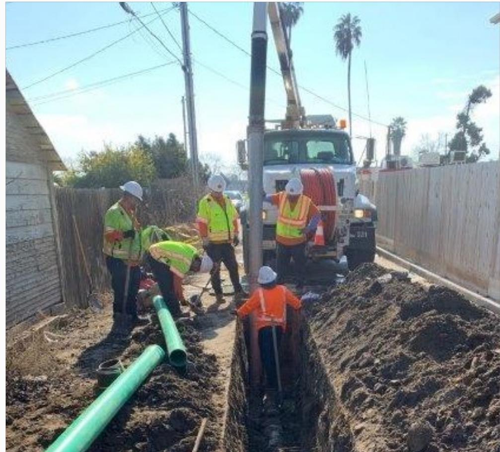
Photo: Workers dig a trench to replace a pipe
