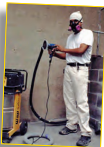
Attach power tools to a HEPA vacuum.
