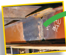
Strip back paint before cutting or welding.
